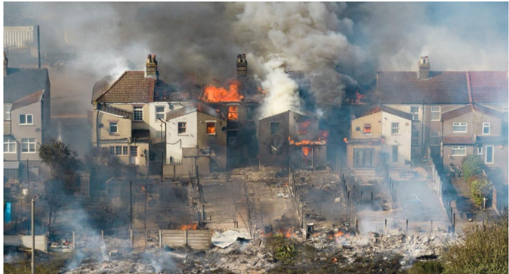
A row of houses on fire in the village of Wennington, Essex © Peter Macdiarmid/LNP
