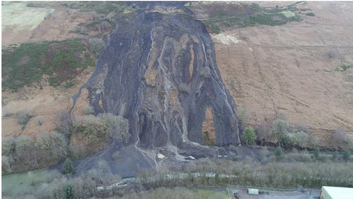
Tylorstown landslip © RCT
